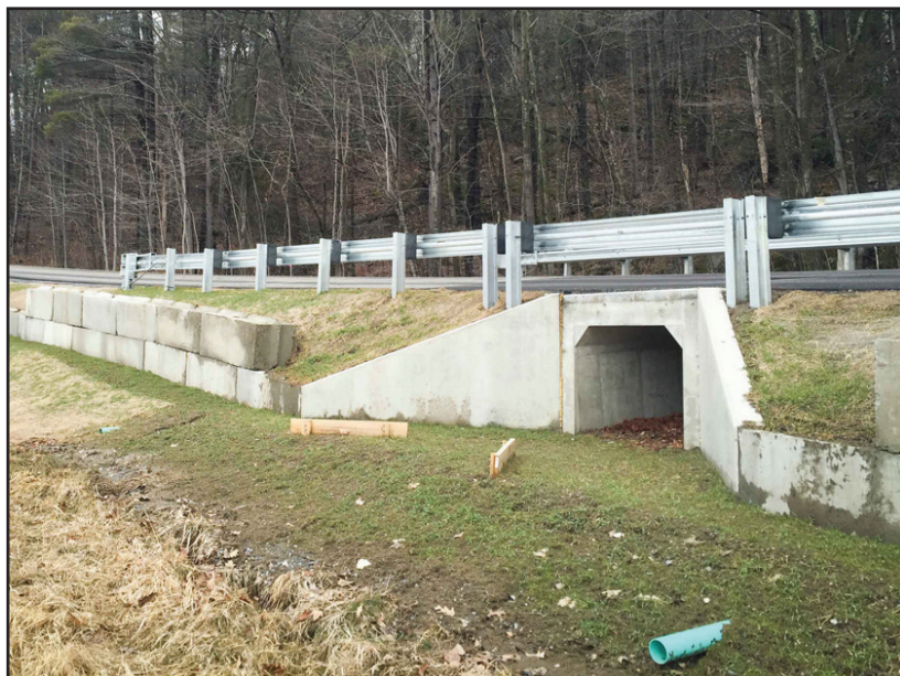
THIS IS ONE of two tunnels that allows amphibians to pass under Monkton Road unharmed during the spring and fall migration seasons. Before the tunnels were built, thousands of amphibian risked death each night crossing from the forest to the swamp.
